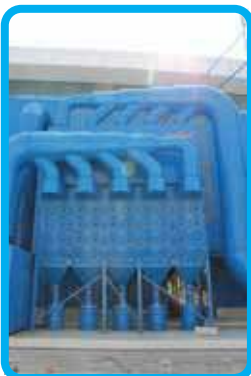
Lead dust treating device, zero pollution
