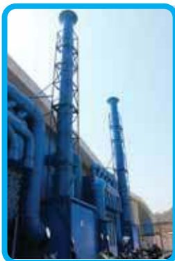
Lead dust treating device, zero pollution
